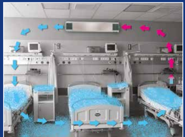
Process of the air treatment with the use of internal UV-C tubes (air)
