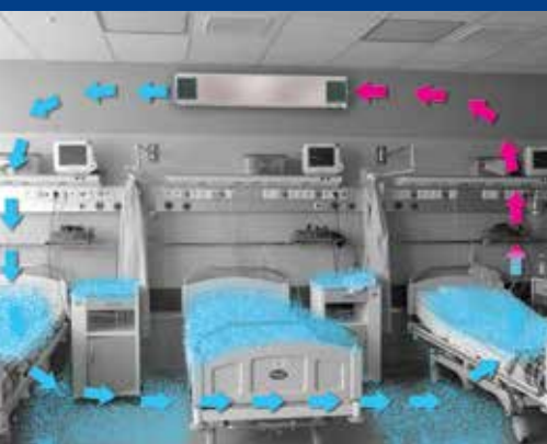
Process of the air treatment with the use of internal UV-C tubes (air)
